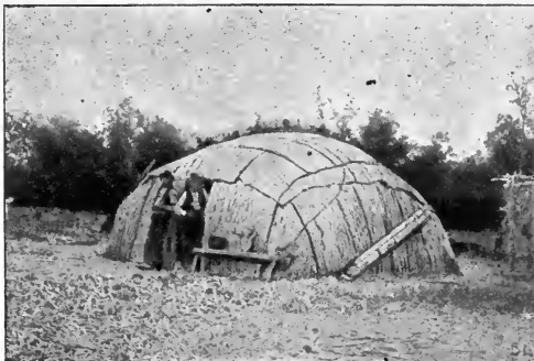
CHIPPEWA BARK HOUSE. (GILFILLAN)
